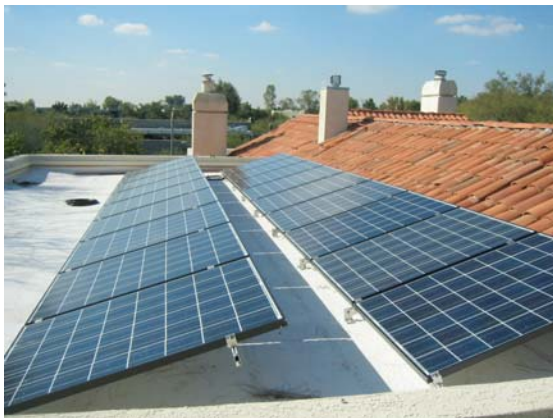
Photovoltaic panels (collectors) hidden behind a parapet wall on a flat roof
